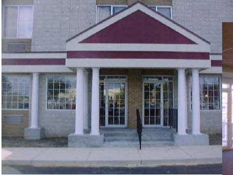
Exterior before Construction
